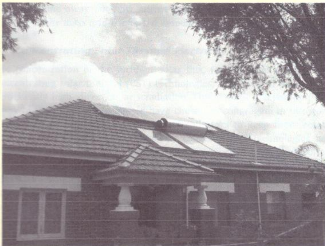
Fig. 5. House with grid-connected photovoltaics and domestic solar water heater.
